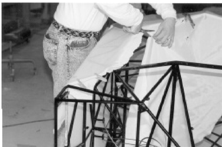
Figure D-2 Fabric Trimmed around Door Opening
