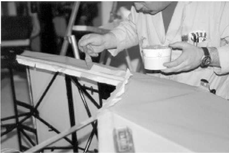
Figure I-5 Finishing Tapes around Door Frame
